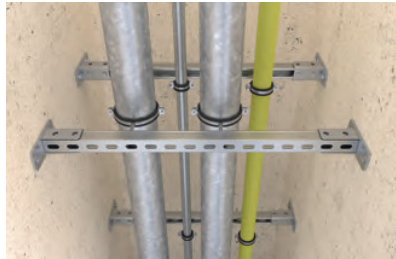
Pipe installation in escape route
